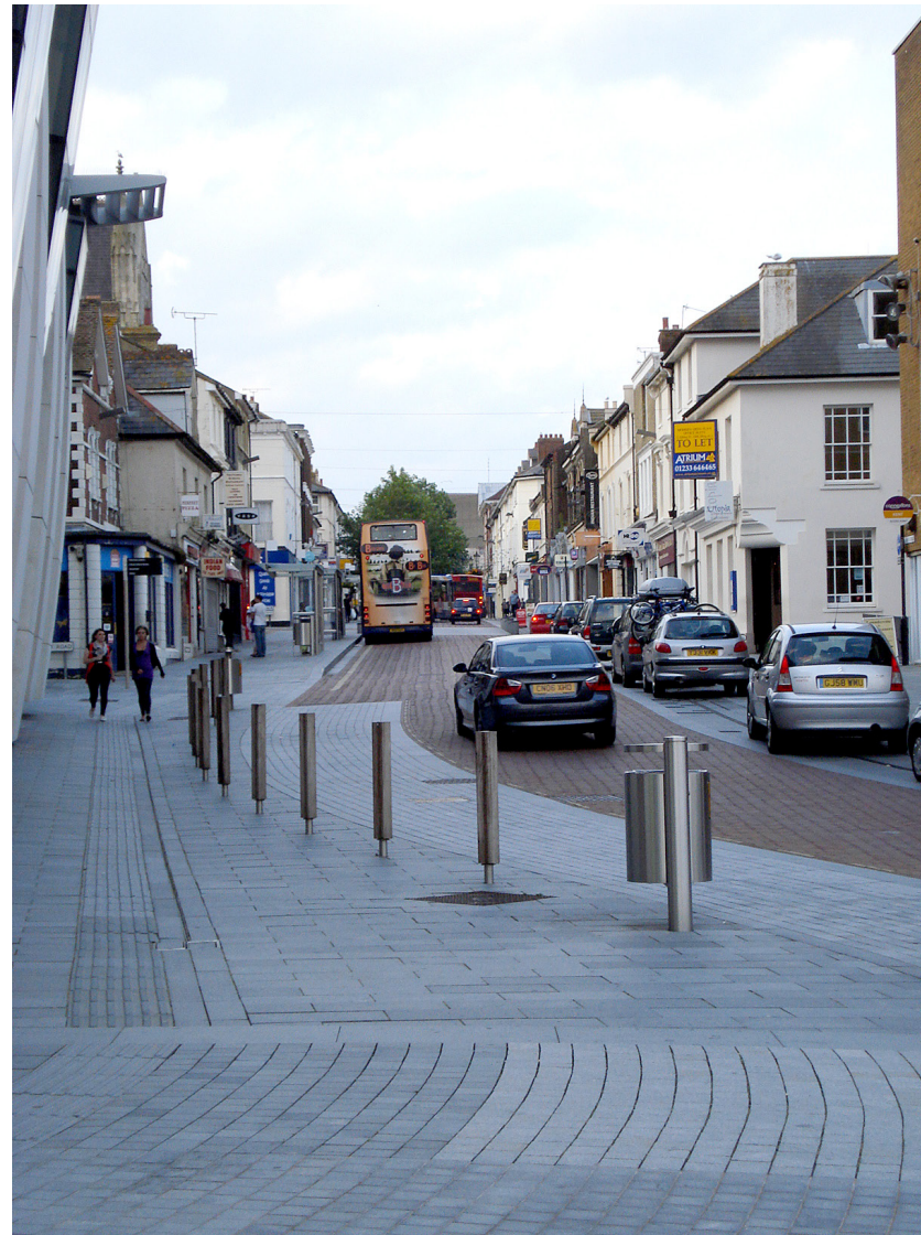
This scheme at Bank Street in Ashford provides a good example the 'less is more' approach to traffic signs
