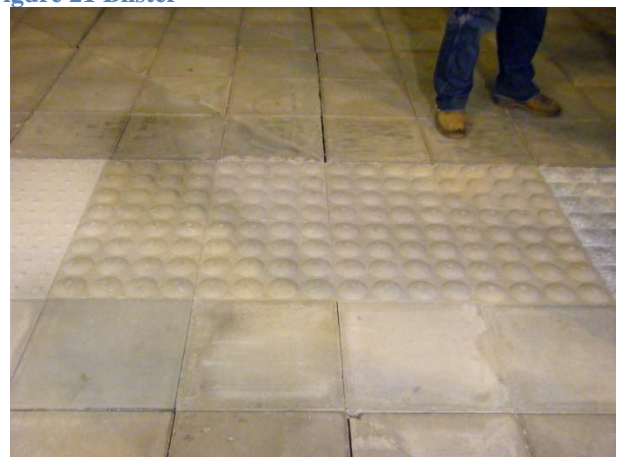
Figure 23 Dome set 15mm above surrounding surface
