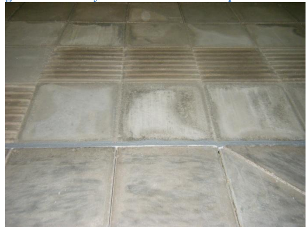
Figure 11 Level Corduroy and non-chamfered 1:8 slope
