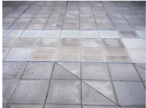
Figure 15 Corduroy on level and on 1:12 slope
