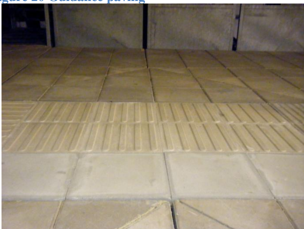
Figure 22 Guidance Paving aligned to cross the road
